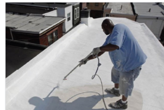
Bioneighbors Sustainable Homes LLC James Peterson of the roofing company BioNeighbors applies a coating of Acrymax to the roof of a row home in Philadelphia
